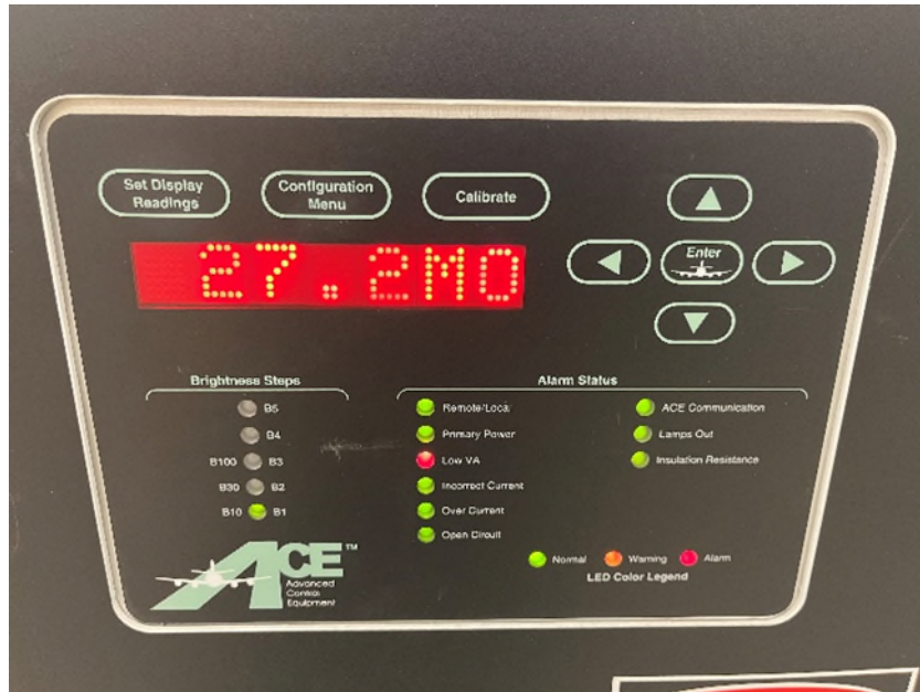
Figures 4 & 5. Two examples of automated Insulation Resistance Monitoring Systems (IRMS)
