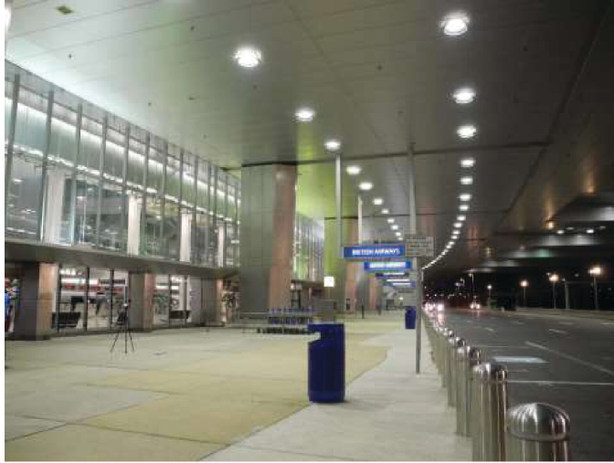
Figure 6-10. Curbside area with deep overhang and a high ceiling.
