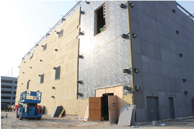
FIGURE 3 A substation was designed to a higher design flood elevation at LGA to alleviate flood risk (Source: Port Authority of New York & New Jersey).
