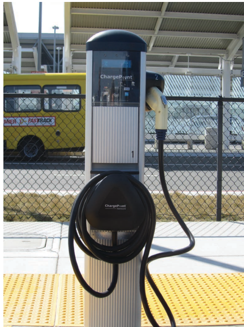
FIGURE 4 Level 2 charging station. (Source: LeighFisher September 2013.)
