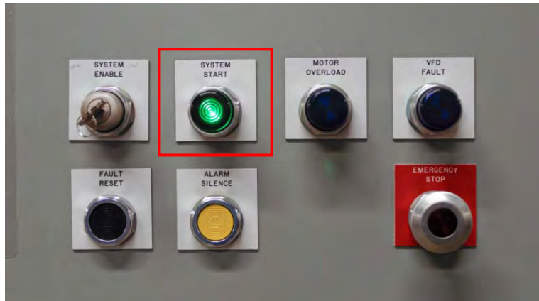
Figure E-26 TURNING THE 'SYSTEM ENABLE' SWITCH OFF
