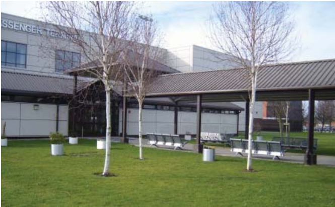
Covered Entry Walkway
