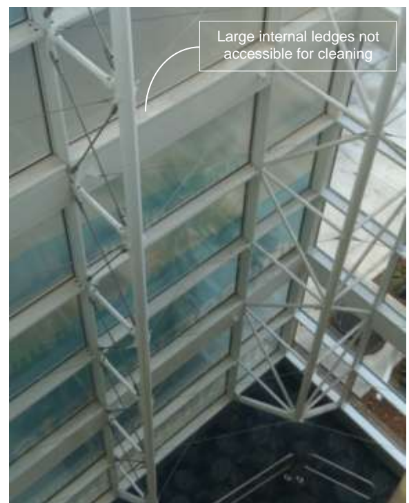
Figure 11: Provide Unobstructed Floor Area for Maintenance and Cleaning of Curtain Wall Framing.
