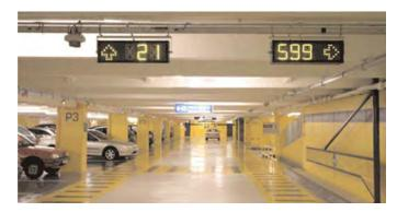
Figure 4.19. Once inside the parking garage, the space management system uses a series of signs to indicate which areas have available parking. Then sensors located above each parking space use red and green indicator lights to inform drivers if a particular space is occupied or not.
