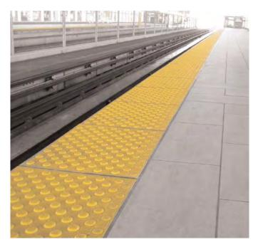
Figure 6.84. Tactile technologies, such as floor dots, can assist the blind from curbside to check-in.
