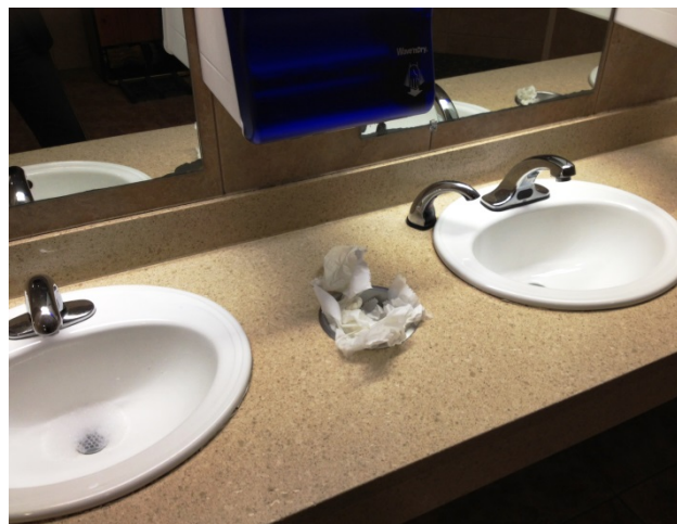
Sloped Trash Container Below Quickly Clogs with Trash
