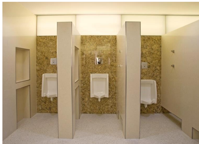
Typical Stall with Thickened Walls Urinals with Thickened Walls Similar to Stalls and Shelf/Alcoves for Belongings
