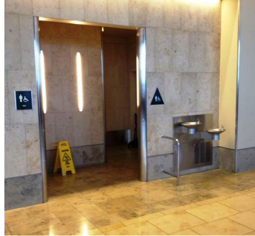
Entrance to Men's – Note California Required Triangular Sign for Vision Impaired
