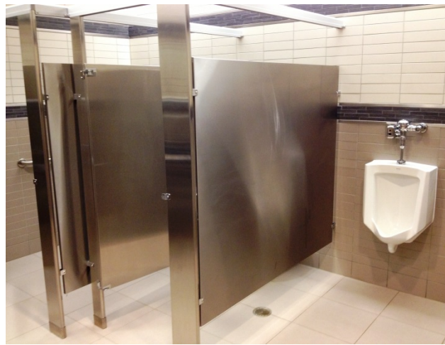
Floor-mounted and Overhead-braced Stalls
