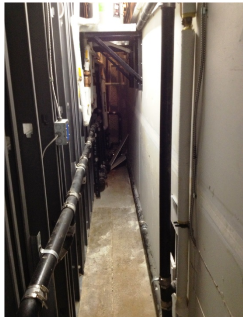
Typical Pipe Chase
