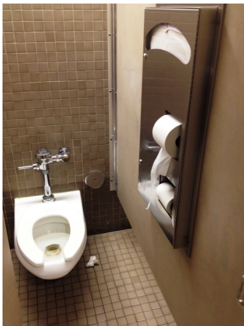
Typical Stall on Older Restroom Set
