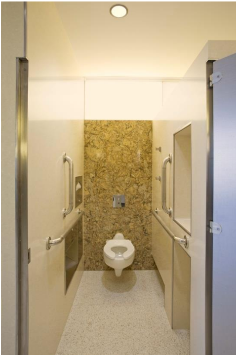
Typical Stall with Thickened Walls Urinals with Thickened Walls Similar to Stalls and Shelf/Alcoves for Belongings
