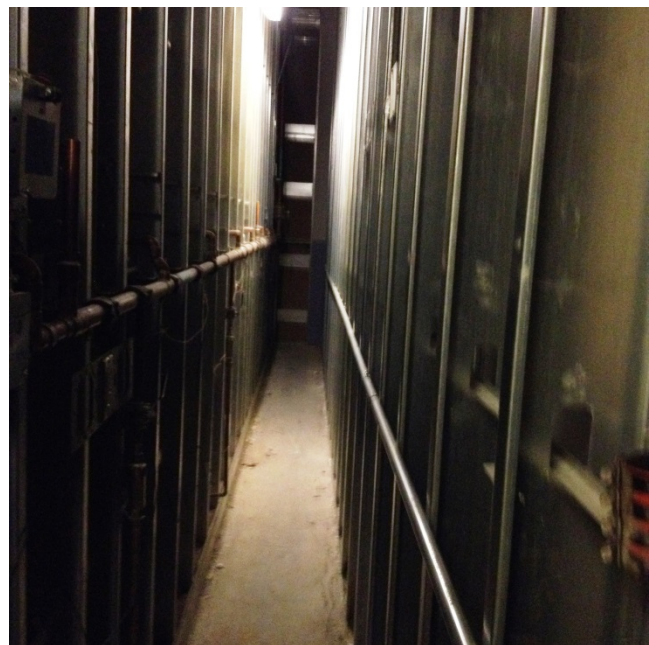
New Pipe Chase with Studs on Concrete Curbs
