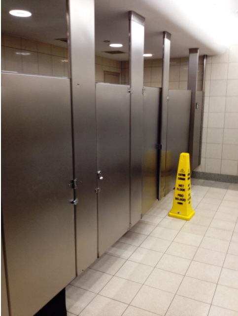
Overhead-braced Stainless Steel Stalls
