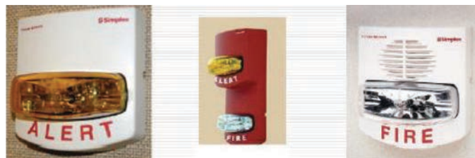
Figure 8-23. Multicolored fire alarm system strobes deployed at Dane County Regional Airport.
