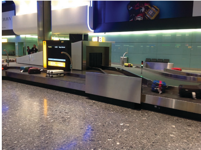
Figure 7-9. Remote-fed flat-plate baggage claim carousel at Heathrow Airport Terminal 2.
